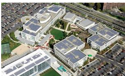
Courtesy: Commercial Scale Installation - eBay
