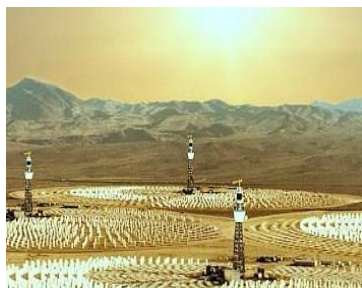
Courtesy: Arizona Solar Farm
