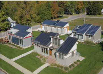
Courtesy: Micro-grid Solar Installation
